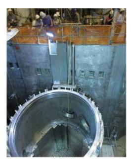
Installing a New Reactor at Watts Bar
